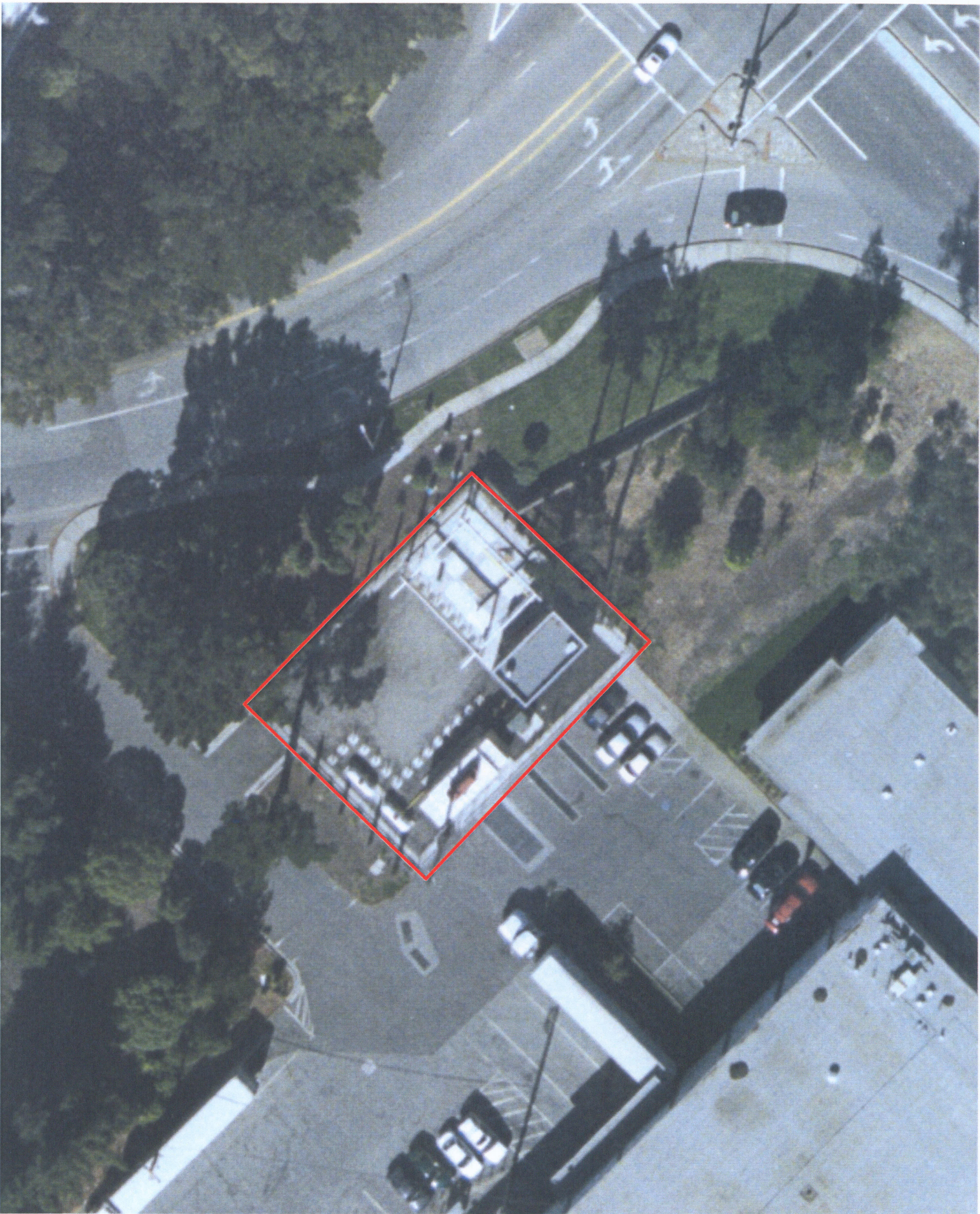
2.b VALLEY DRIVE LIFT STATION
